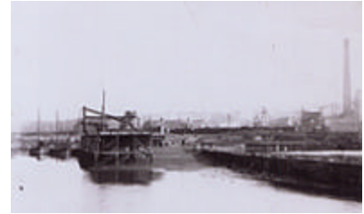
Landward view of Morrison's Haven Harbour with Prestongrange Colliery in the distance
