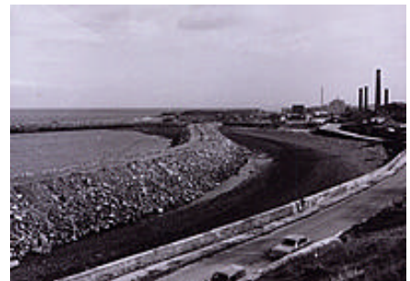
Land Reclamation at Morrison's Haven, c1952
